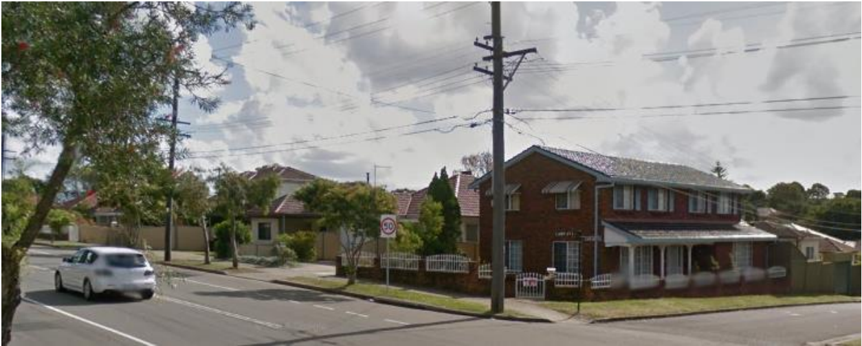
Picture 1 – North side of Amy Street looking west of Smith Street
