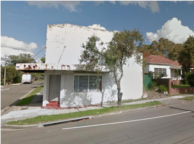
Figure 3 – Amy Street Streetscape
