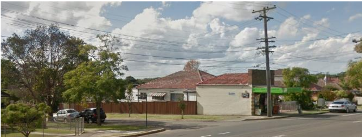
Picture 2 – North side of Amy Street looking east of Maunder Street
